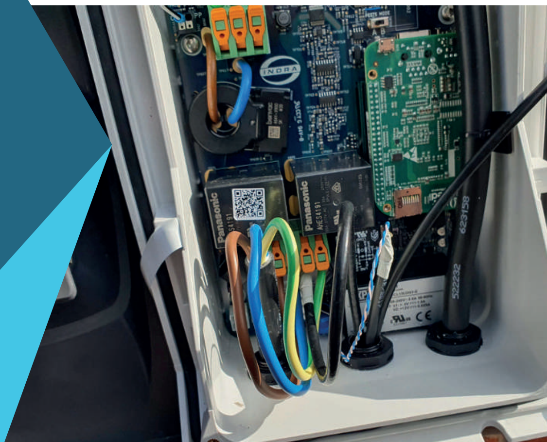
Images of 'pig-tailed' mains cables into the charger unit.
